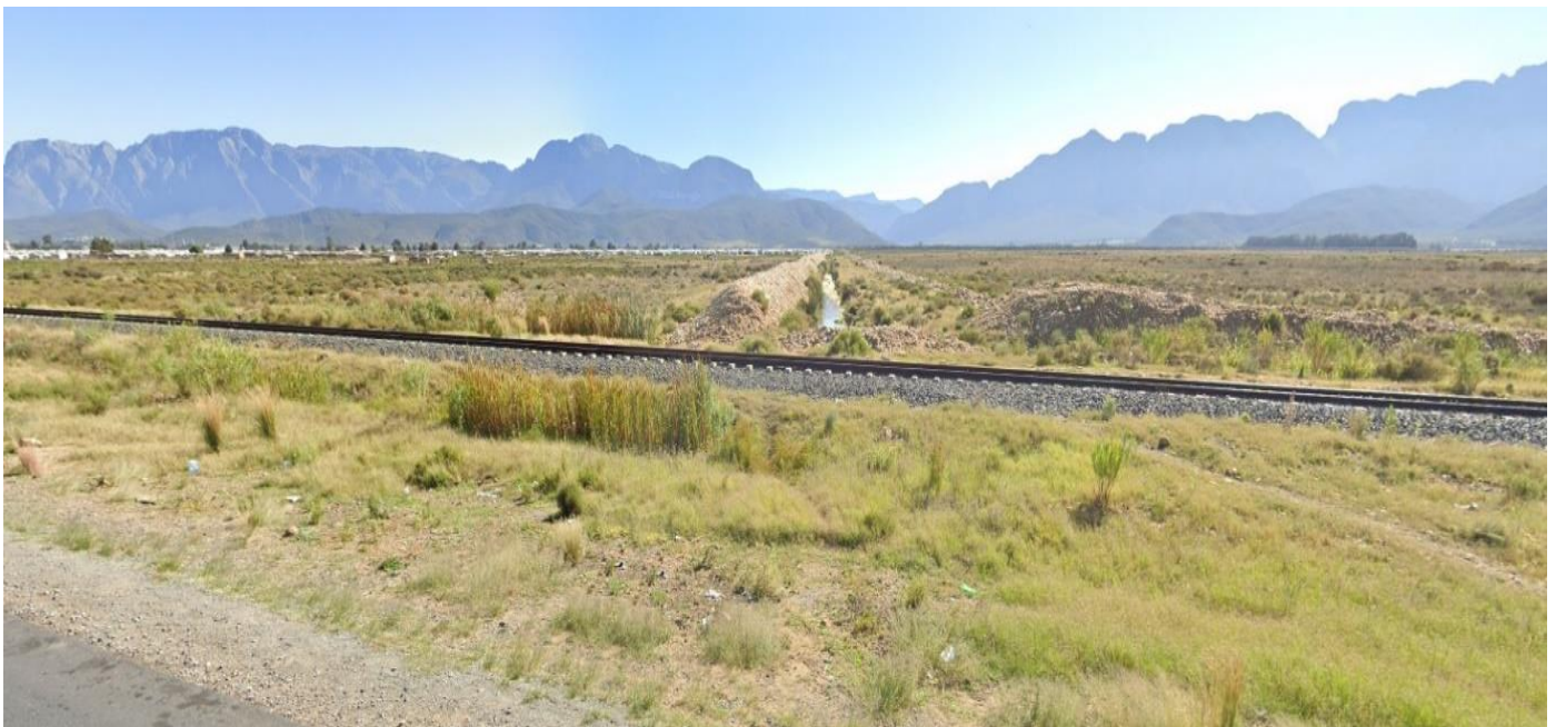
Figure 2: Drainage furrow (1.6 km outside Worcester and 1 km before Overhex Cellar), which runs northwards in the direction of the Hex River Valley.
